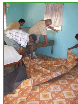
BIWG installing floor covering
